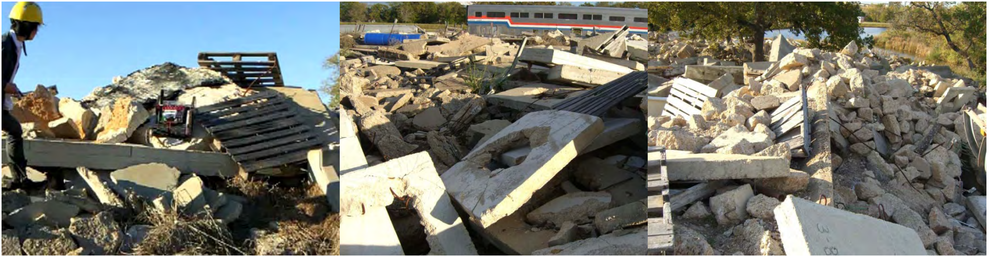
Traverse of RC rubble pile (40 m x 40 m)
